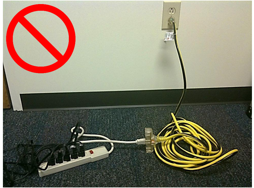
Improper power strip use: plugged into extension cord. Power strips must be plugged directly into an outlet; extension cords are for short term use only.
